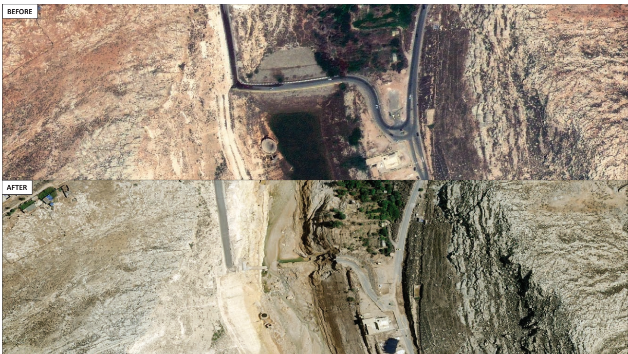
Figure 2: Abu Mansour Dam
