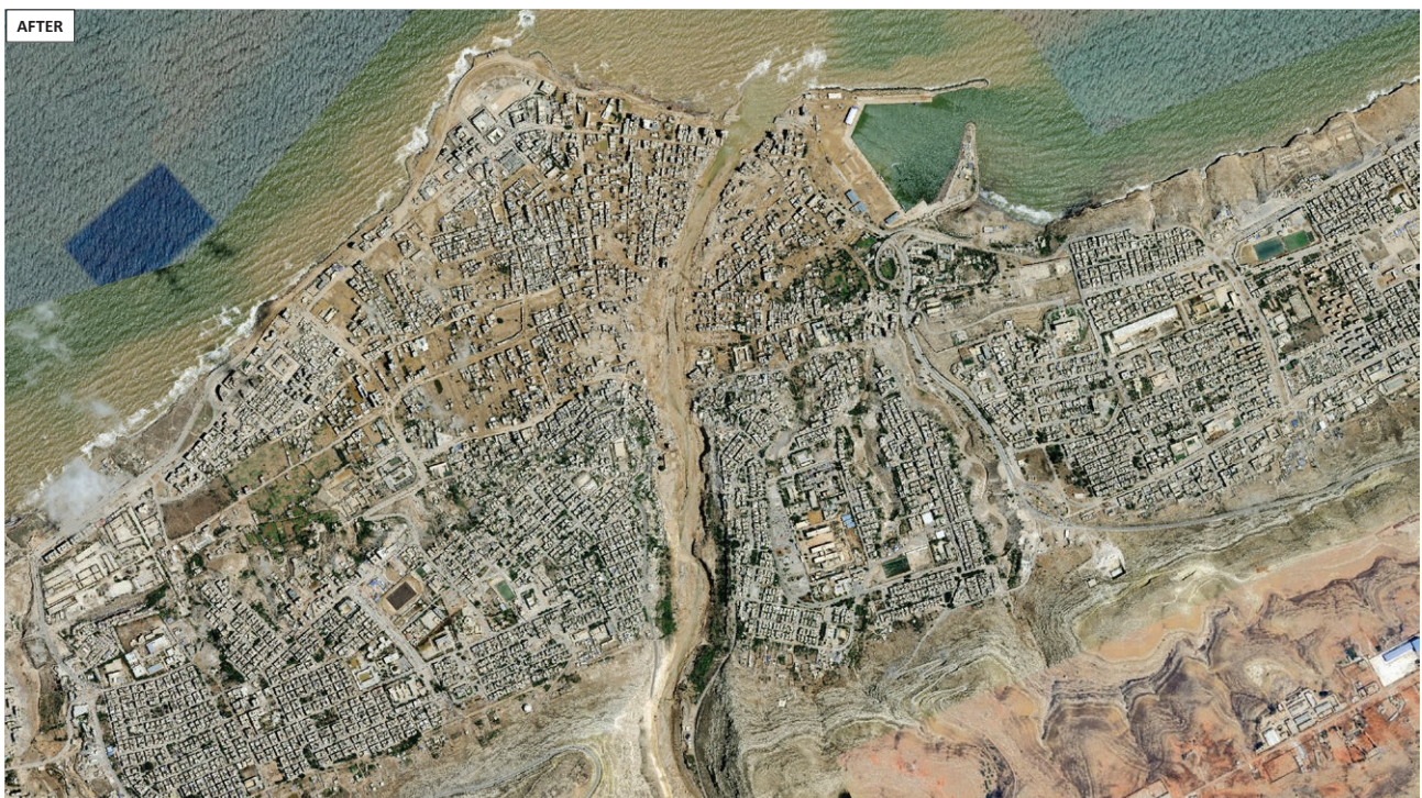
Figure 8: Derna City Following the Floods (13SEP2023)
