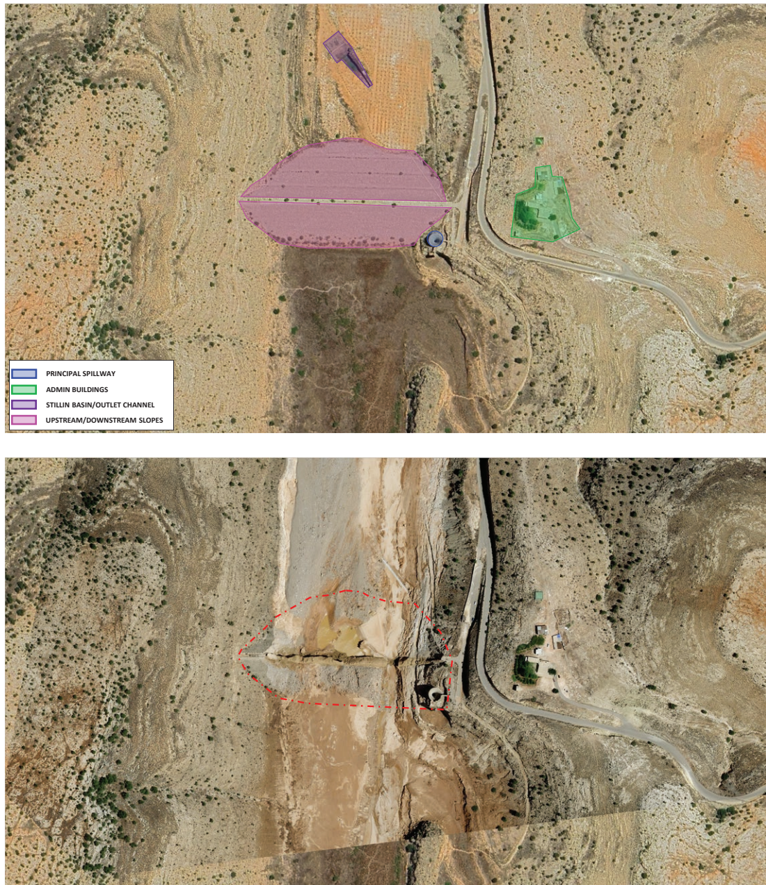
Figure 45: Bou Mansour Dam Prior (Left) and Post (Right) Flood
